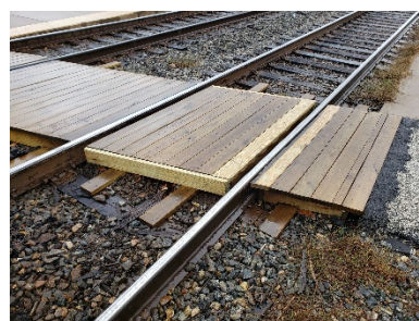
Repairs to pedestrian crossing at Quantico
