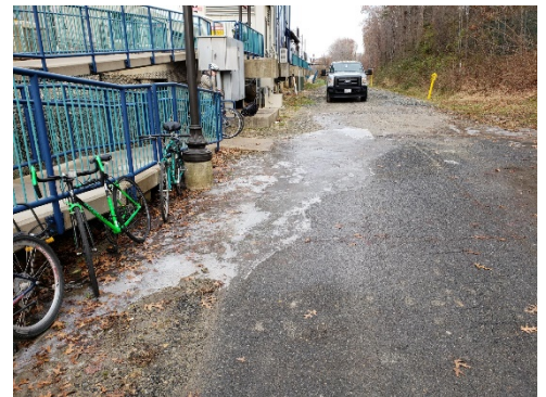
Ice Problem Before Drainage Ditch Reestablished at Franconia-Springfield
