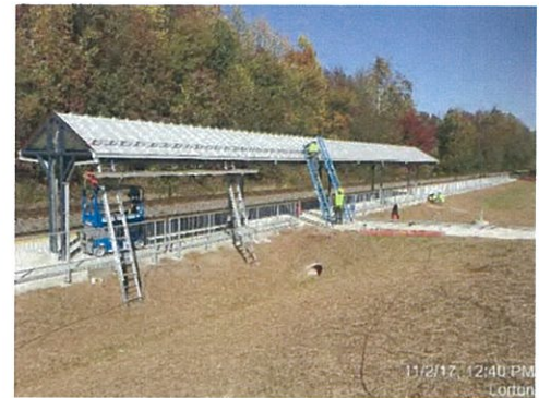
The finished roof is applied to the canopy steel over the platform extension at Lorton
