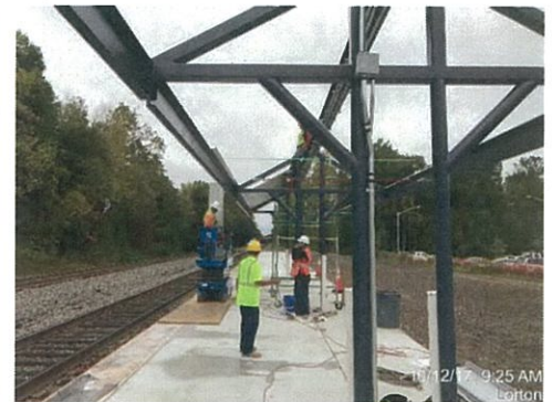
Workers erect canopy steelover the platform extension at Lorton Station.
