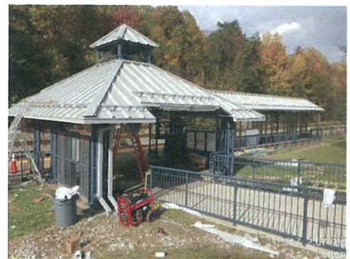
Roofing and drainage gutters are replaced on the existing canopy at Lorton as part of the platform extension project.
