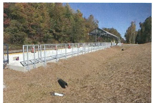
New railings are mounted to the edge of expanded platform at Lorton.
