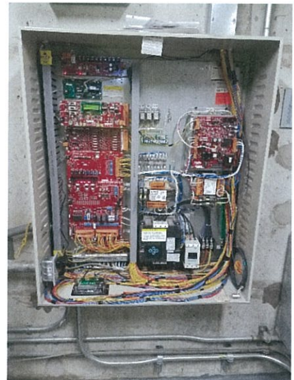
Franconia-Springfield West Elevator Modernized Control Center
