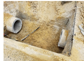
Drainage pipe repairs at the Leeland Road Station.
