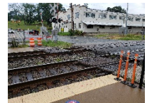
Repaired timber pedestrian crossing
