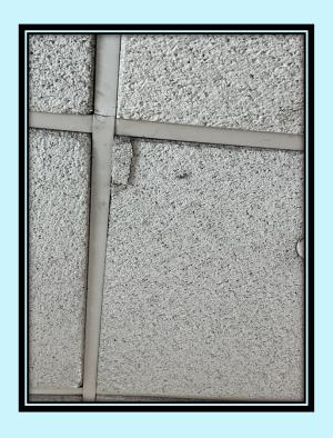
Ceiling tile and grid have been improperly repaired and adjusted.
