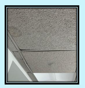
Ceiling Tiles are ill-fitted to the grid.
